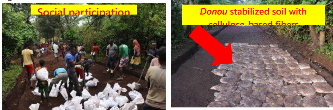
Figure 3: Community participation in constructing small-scale roads with improved donou technology.
